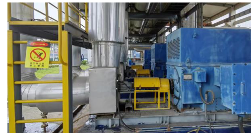
Improvement of Chilled Water Pumps
